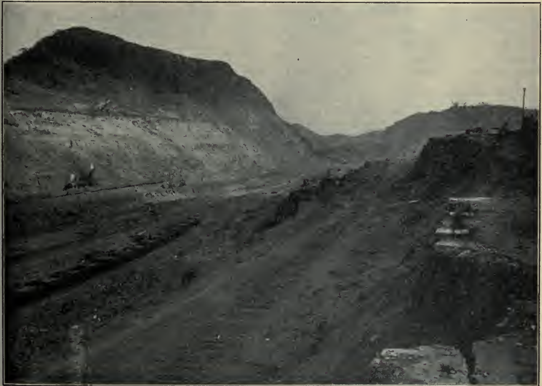
FIG. 326. — A view along the Canal route, in 1909. When this great cut in the earth is deep enough, it will be flooded with water and large ocean ships will then sail through it.
